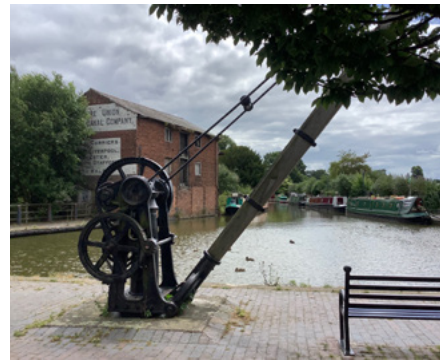
Decaying Shropshire Union Canal Company building and crane, Ellesmere Wharf, on the Llangollen Canal
